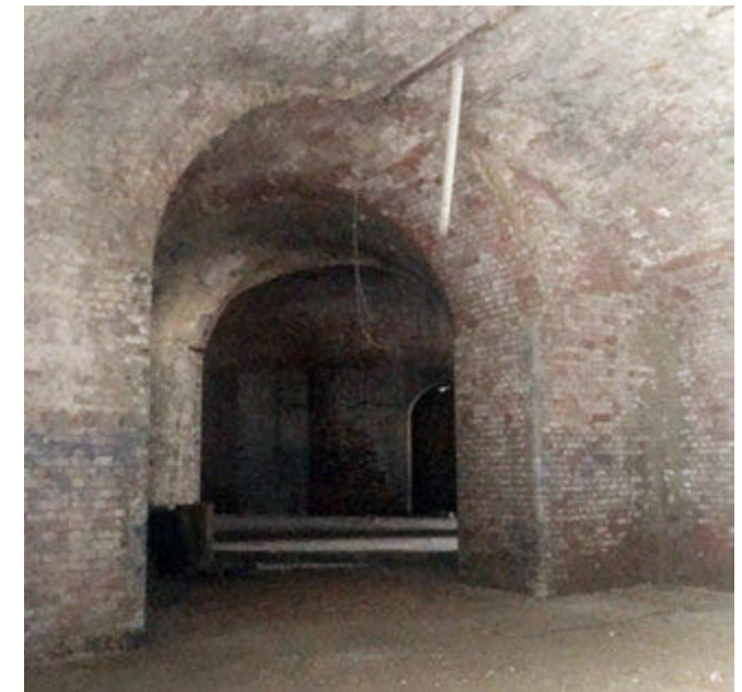
Fig 5.3.18: Existing brick vaults which will house the gallery space.
