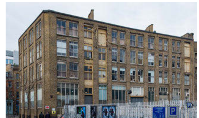
Fig 5.5.17: Shoreditch Precedent - Recessed Brick Panels
