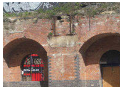
Fig 5.4.10: Visible 'I' beams of historic structure
